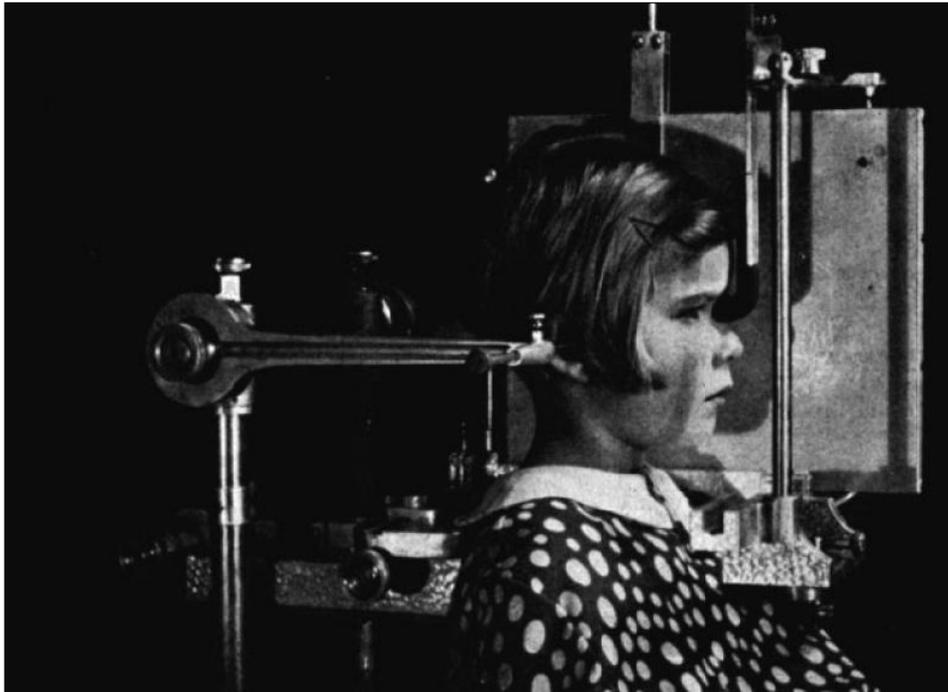
Fig. 13 The child's head adjusted to the head holder. Note the cassette in place for the lateral roentgenogram.
