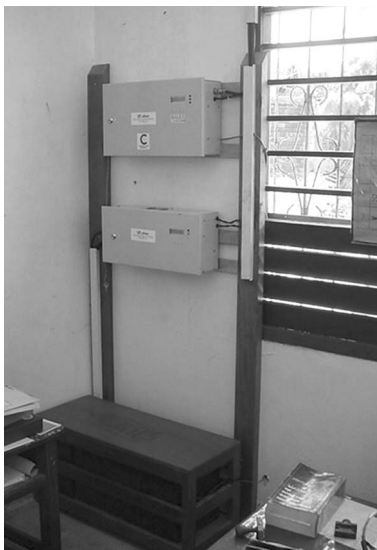
Fig. 8. Solar modules and communication tower in the HP of Lago Cuipari.
