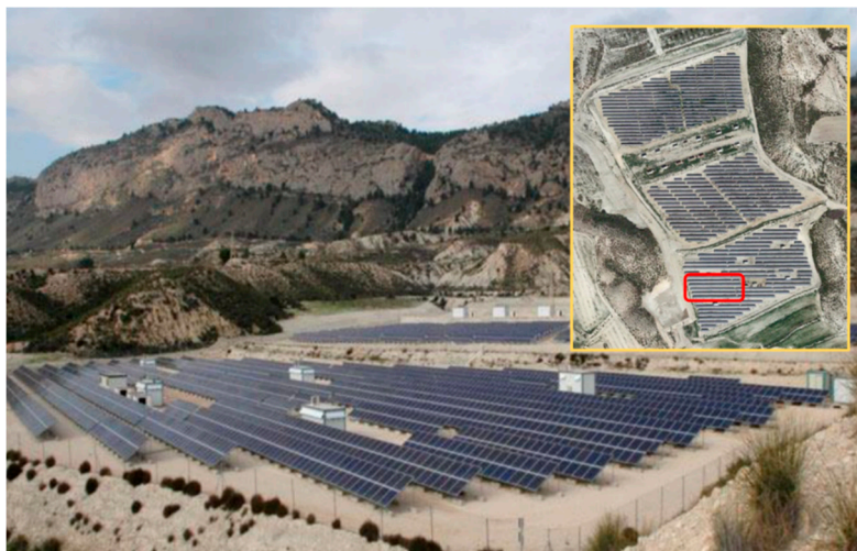
Figure 3. The 2.12 MW p Yéchar photovoltaic plant (Murcia), in the inset the sector of modules which have been monitored using thermographic camera is shown.
