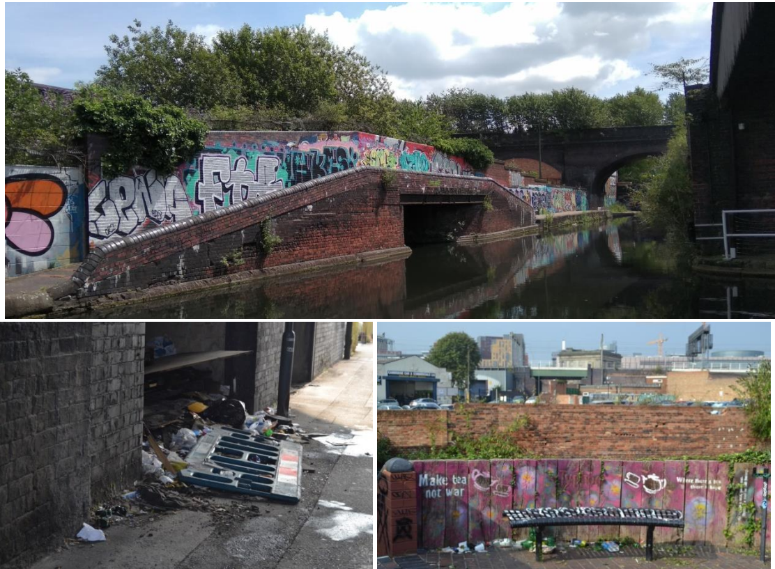
Figure 9. Digbeth and signs of vandalism, deterioration and dirt. Source: Author, 2019, 2018 and 2020.
