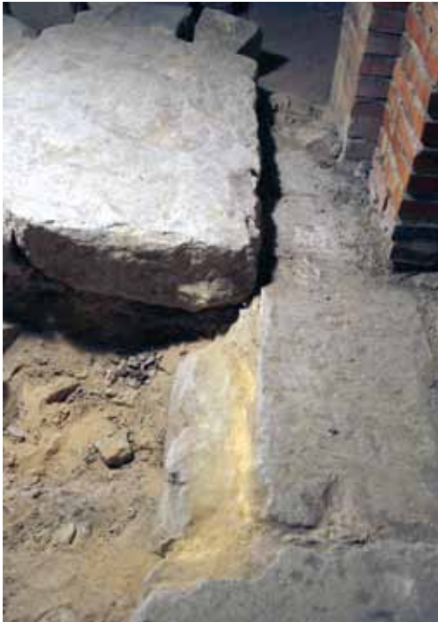
ILLUSTRATION 8. SANTO DOMINGO DE SILOS: NORTH WALL OF THE LOW CHURCH: DETAIL OF THE RECESS, BASE OF THE BLIND ARCHES AND FOUNDATION OF THE TOWER (PHOTO: FÉLIX PALOMERO).
