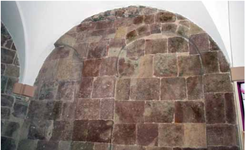
ILLUSTRATION 14. SANTA MARÍA DE VILLAVELAYO: BLIND ARCHES THAT RUN ALONG THE SOUTH WALL. (PHOTO: FÉLIX PALOMERO).
