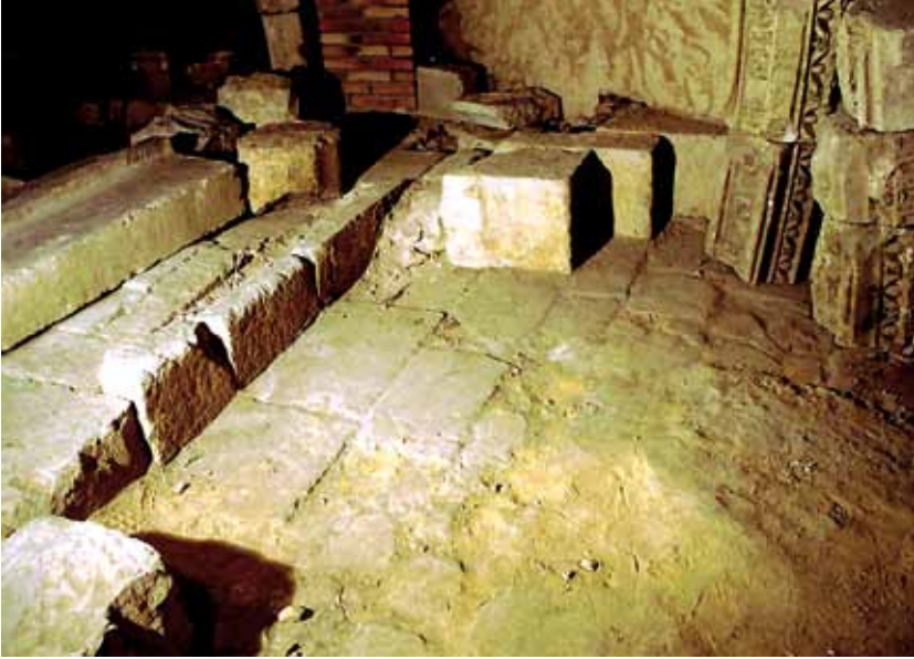
ILLUSTRATION 7. SANTO DOMINGO DE SILOS: NORTH WALL OF THE LOW CHURCH, FLOOR OF THE ATRIUM AND BASE OF THE DOORWAY ADDED IN THE MID-12 TH CENTURY (PHOTO: FÉLIX PALOMERO).
