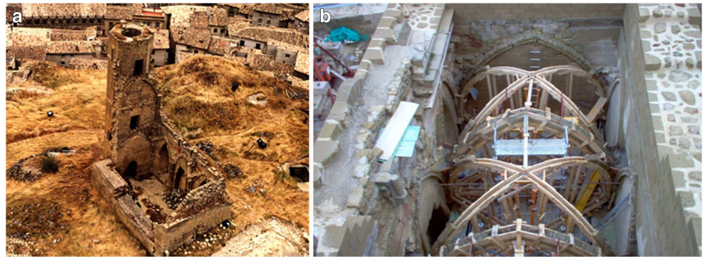
Fig. 3 Pedro Palace before (a) and during the restoration work (b)
