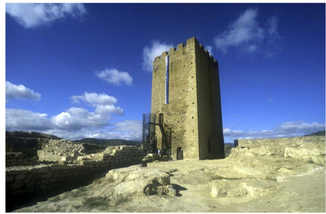
Fig. 2 The Homenaje Tower after the restoration
